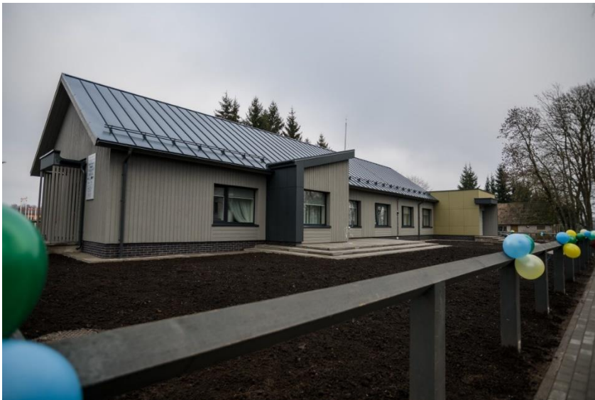
Construction of an orphanage in Lithuania with the help from clubs from Nothern Germany, LCIF and NSL. A project by 111NB, Germany.
